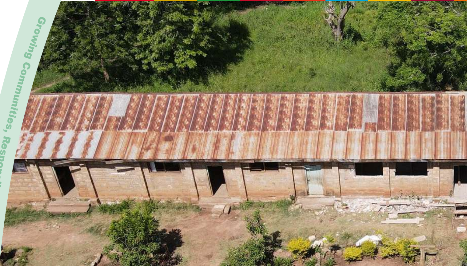
Kakuzi Primary School before renovation.
