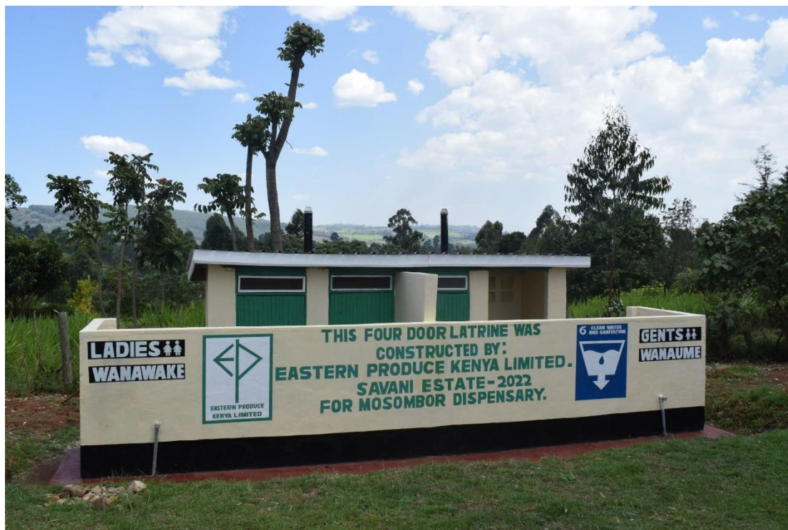
Photos showing a constructed 4 door sanitation facility at Mosombor Dispensary
