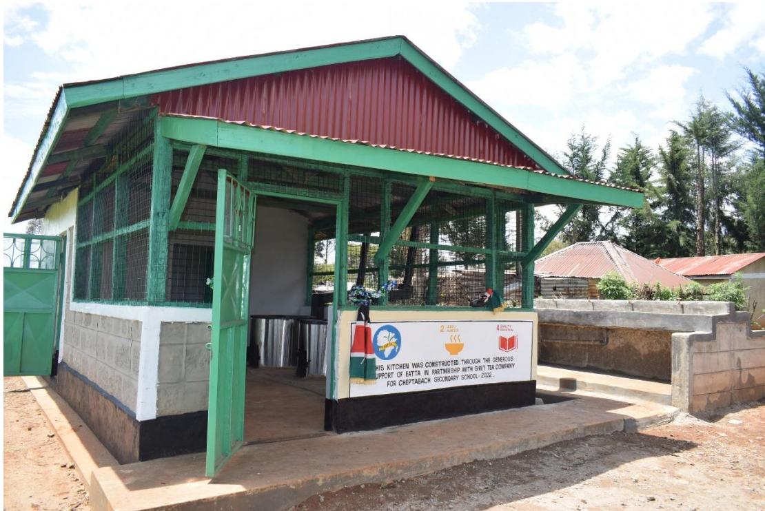
Photo showing the constructed school kitchen and adjacent to it a dishwashing/handwashing basin
