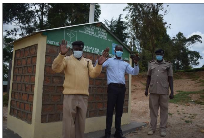
Photo showing a sanitation facility constructed and handed over to Kosoiywo Chief's Office
