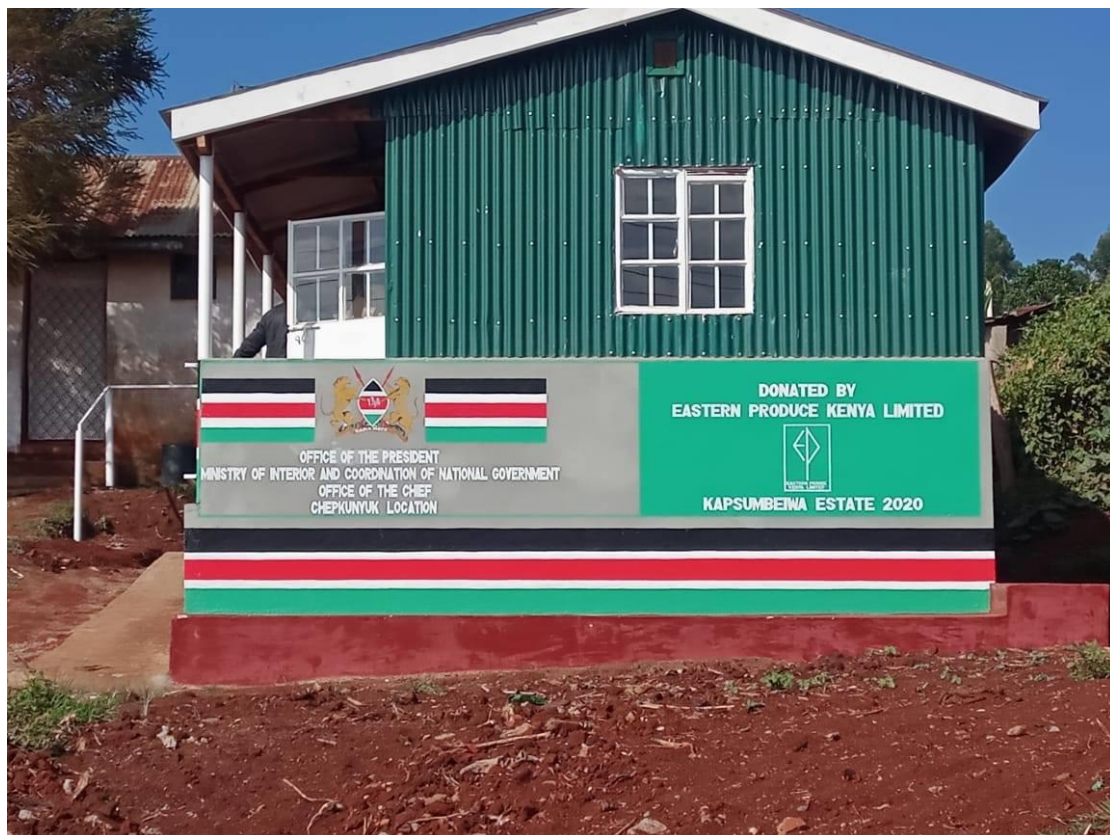
Photo showing constructed Chepkunyuk's location office
