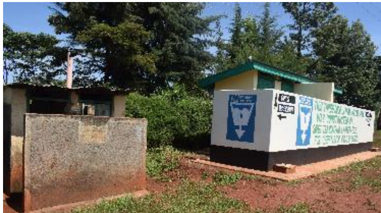
Photo showing a 4 door sanitation facility constructed and handed over at Cheptababach Primary School. Besides it, the previous facility utilised by the school.
