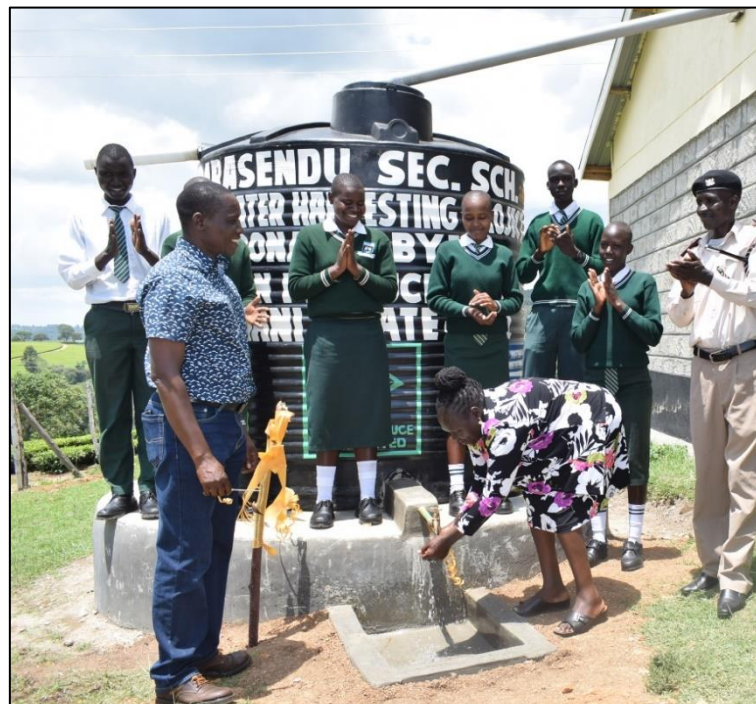
Photo showing A rain water Harvesting System Installed at Barasendu Secondary School
