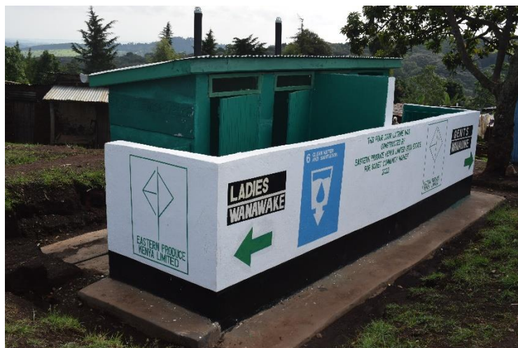
Photo showing a constructed double door latrine being handed over to Tendwet primary school
