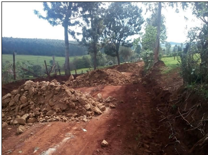
Photo showing Work in progress at Cheptabach Road in June, 2019
