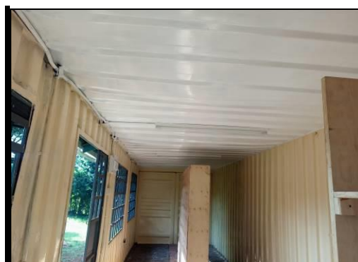
Ongoing works at the site
