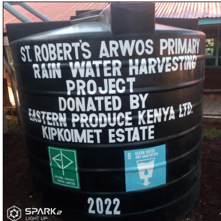
Photo showing a Rain Water Harvesting System Installed at St Robert's Arwos Primary School.
