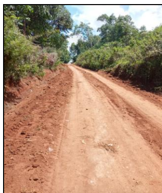
Photo showing Siret- Temso Road
