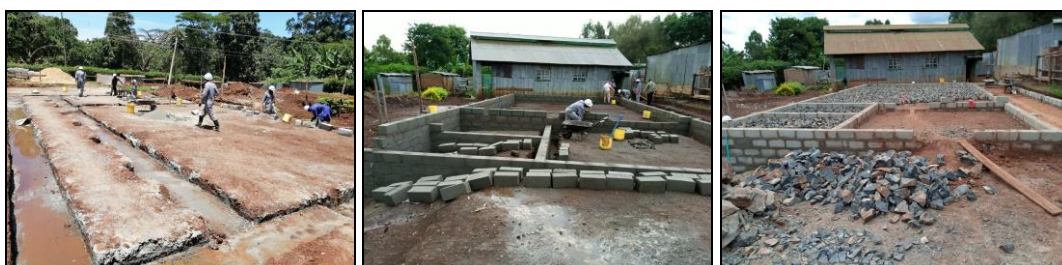
Photos showing work in Progress at Savani secondary School
