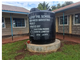
Photo showing installed Rain water harvesting kit at Soiyet Primary School
