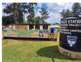
Photo showing a 3 door + urinal Sanitation Facility constructed at Nandi Hills Police Station
