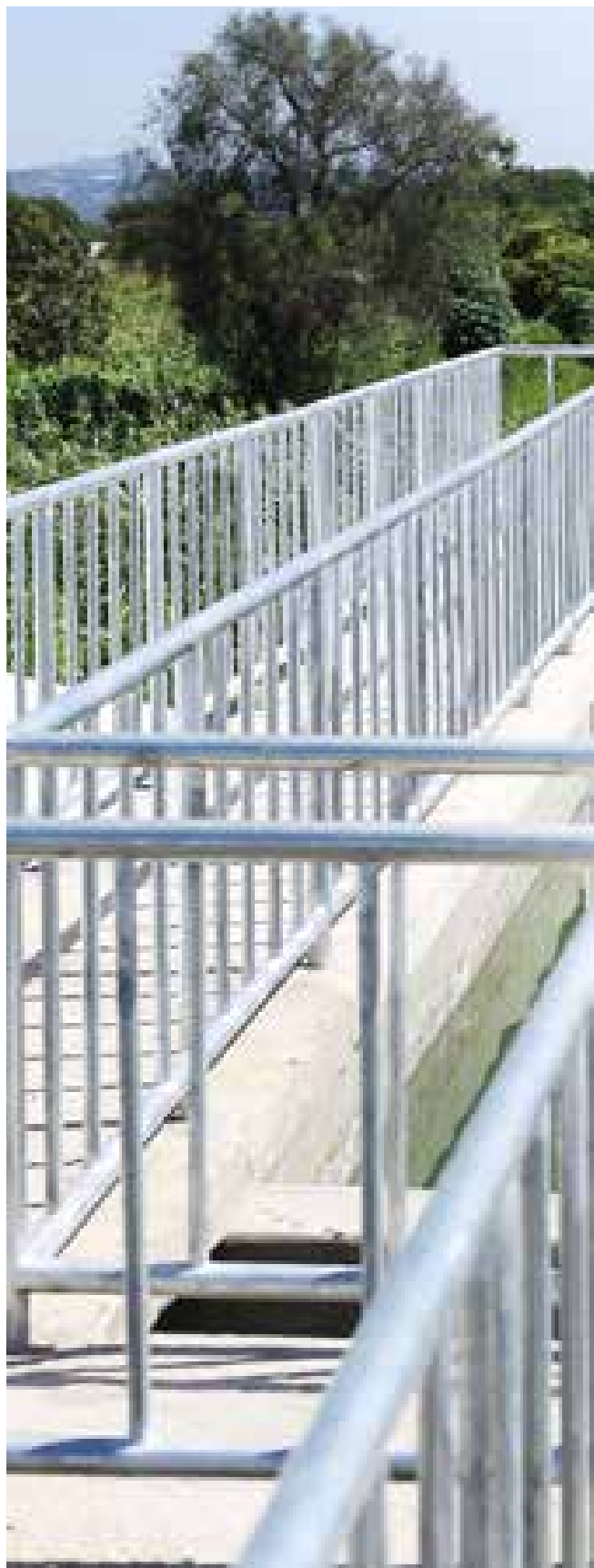
SBL's Nalgonda Water Treatment Plant at Basuto in Manyara Region
