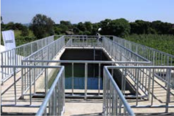
SBL's Nalgonda Water Treatment Plant at Basuto in Manyara Region
